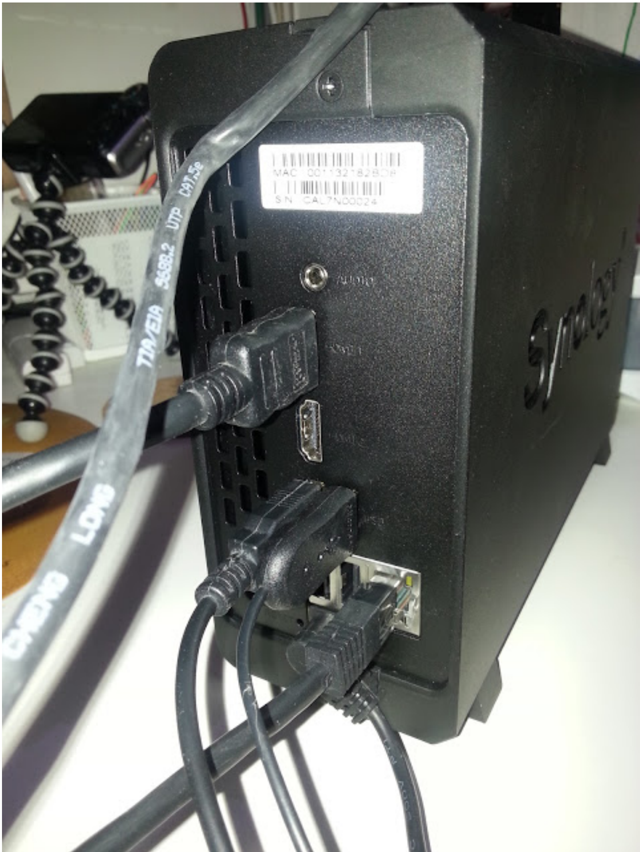
Configuration de Surveillance Station
